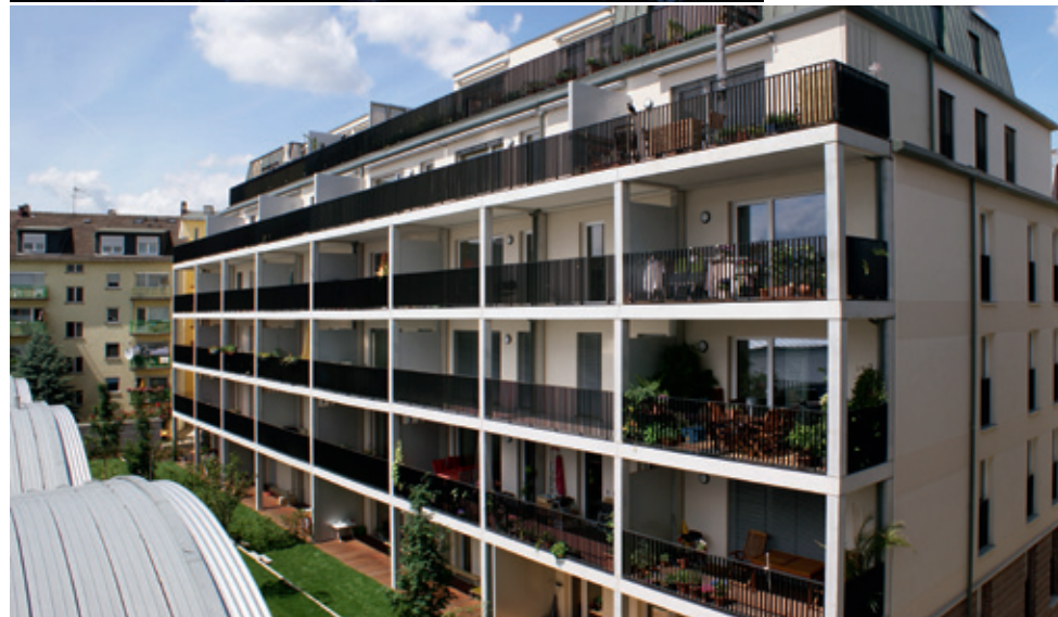
Above: A comprehensive remodelling of a former tram depot in Frankfurt am Main introduced 11 townhouses, with a total of 156 apartments, all built to passivhaus standards.
